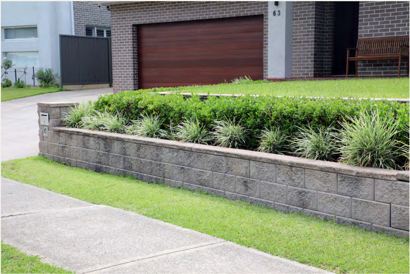
Example of retaining wall and private landscaping
