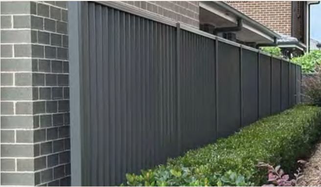
Example of boundary fence
